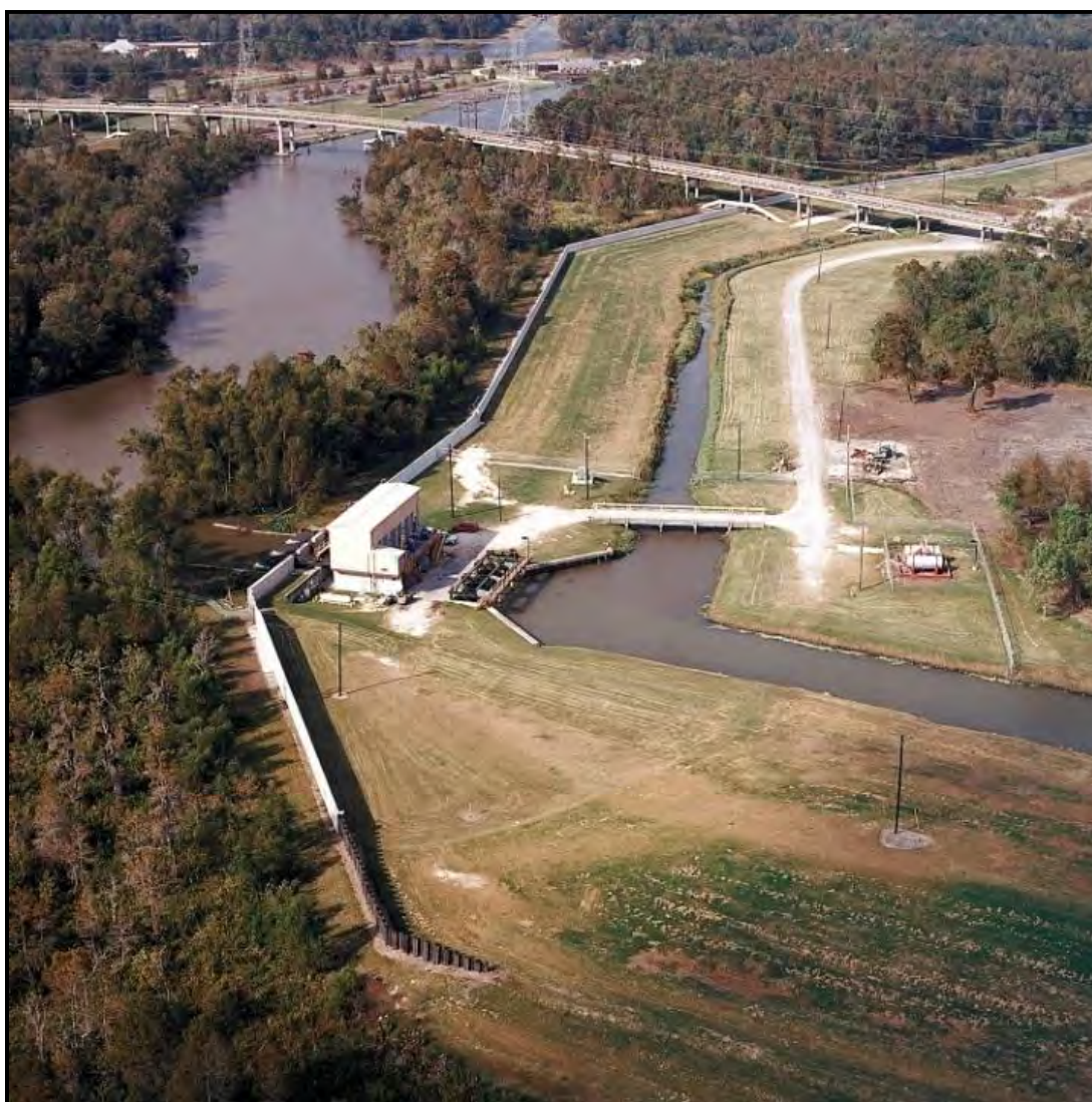
Figure 2-3. Aerial photo showing line-of-protection and associated interior drainage facility.
